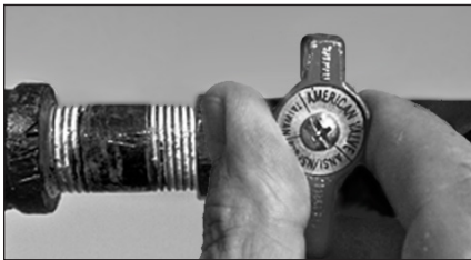
Figure 45 - Gas valve in "off" position.
