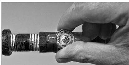
Figure 49 - Gas valve in "on" position.
