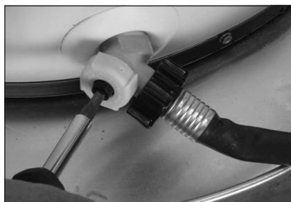
Figure 20 - Draining the old water heater.
