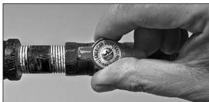
Figure 31 - Gas valve in "on" position
