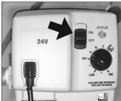
Figure 37 - Turn gas control/temperature knob OFF.
