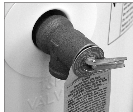
Figure 24 - Temperature and Pressure Relief Valve
