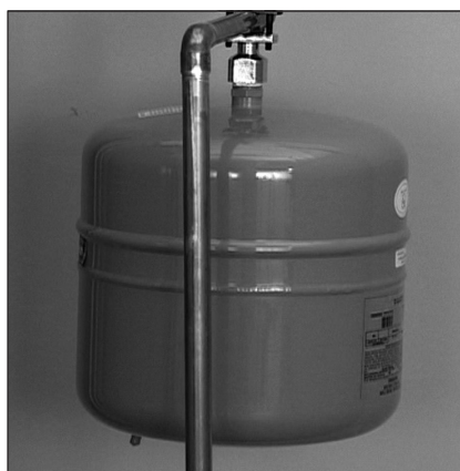
Figure 28 - The Thermal Expansion Tank should be pressurized with air, using a hand pump, to match the home's incoming water pressure.
