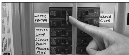
Figure 42 - Circuit Breaker.
