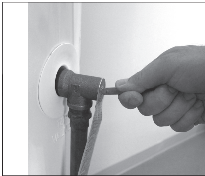
Figure 49 - T&P Relief Valve.
