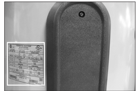
Figure 22 - The water heater’s electrical requirements can be determined from the data plate.
