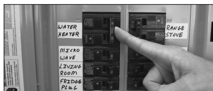
Figure 35 - Circuit Breaker.
