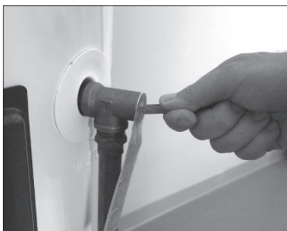
Figure 41 - T&P Relief Valve
