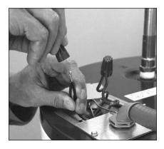
Figure 19 - Connecting the electrical wires.
