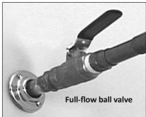
Figure 17 - Fully open the cold water supply valve.
