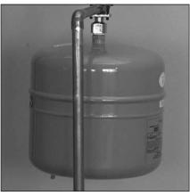
Figure 16 - The Thermal Expansion Tank should be pressurized with air, to match the home's incoming water pressure.
