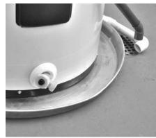
Figure 6 - A suitable drain pan piped to an adequate drain can help protect flooring from leaks and drips.
