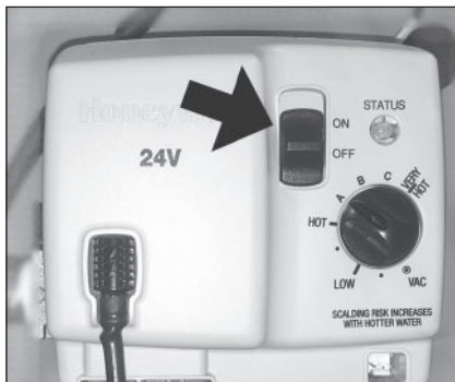
Figure 37 - Turn gas control/temperature knob OFF.
