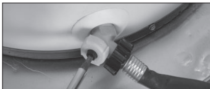
Figure 39 - Draining the water heater.
