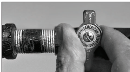
Figure 45 - Gas valve in "off" position.
