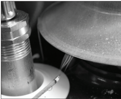
Figure 34 - Test the air supply and vent to make sure the water heater has adequate air and is venting properly.
