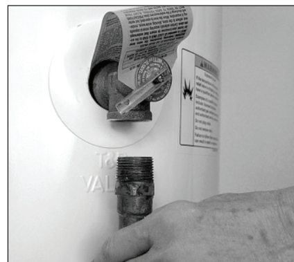
Figure 21 - Removing the T&P Relief Valve discharge pipe.
