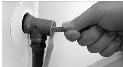
Figure 42 - T&P Relief Valve.
