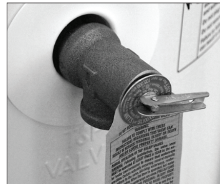
Figure 24 - Temperature and Pressure Relief Valve
