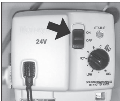
Figure 44 - Turn the gas control valve off.
