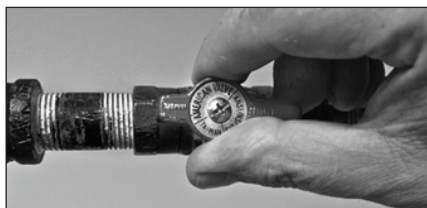
Figure 31 - Gas valve in "on" position
