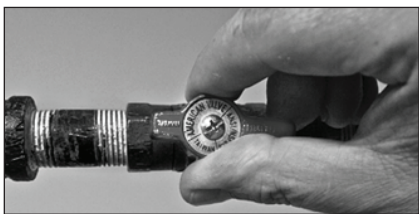
Figure 49 - Gas valve in "on" position.
