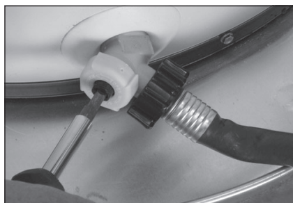
Figure 20 - Draining the old water heater.
