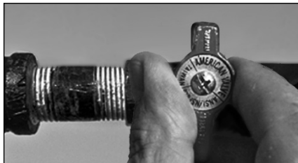
Figure 46 - Gas valve in “off” position.
