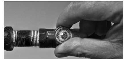
Figure 50 - Gas valve in “on” position.
