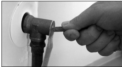
Figure 42 - T&P Relief Valve.
