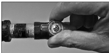
Figure 31 - Gas valve in "on" position
