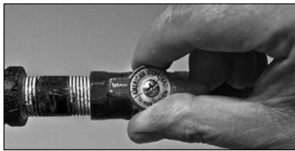
Figure 49 - Gas valve in "on" position.
