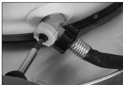
Figure 20 - Draining the old water heater.
