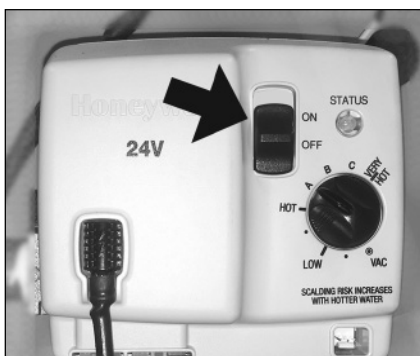
Figure 44 - Turn the gas control valve off.
