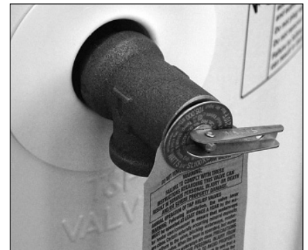
Figure 24 - Temperature and Pressure Relief Valve
