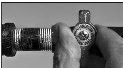
Figure 45 - Gas valve in "off" position.
