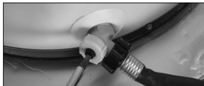
Figure 39 - Draining the water heater.
