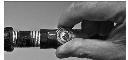
Figure 58 - Gas valve in “on” position.
