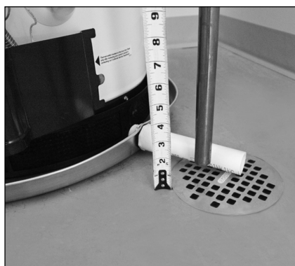
Figure 26 - Temperature and Pressure Relief Valve Pipe
